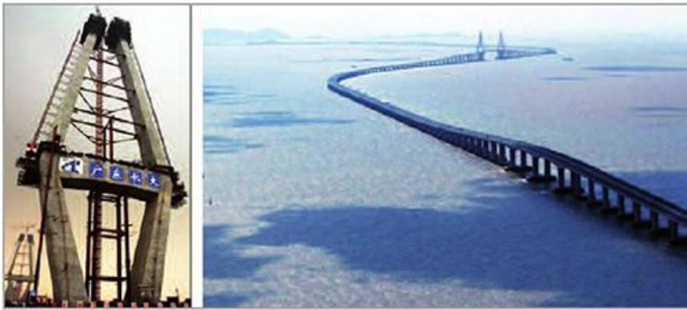
Figura 15 - Hangzhou Bay Bridge.
